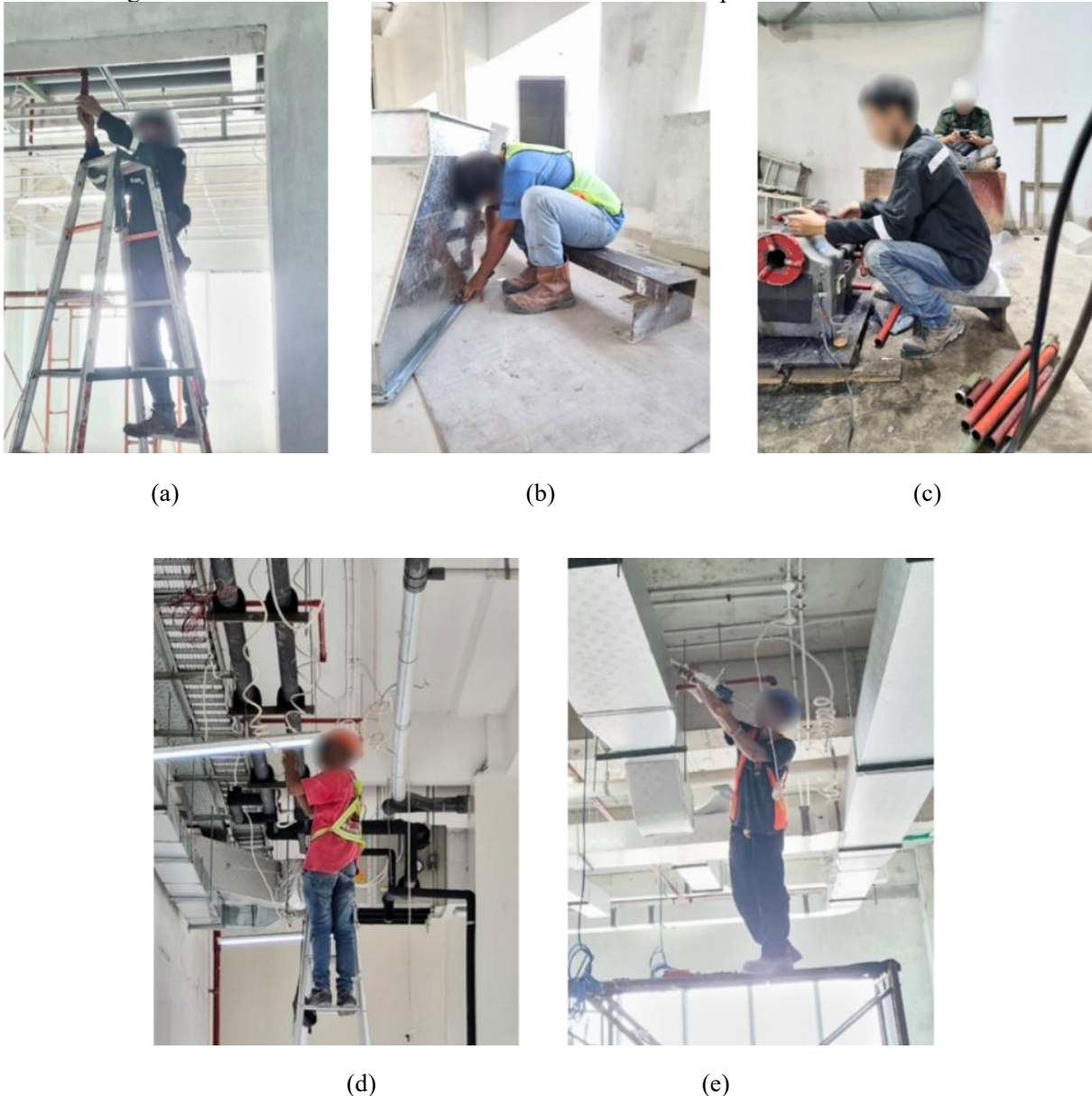
Figure 1: Various Construction Work for Hospital X
